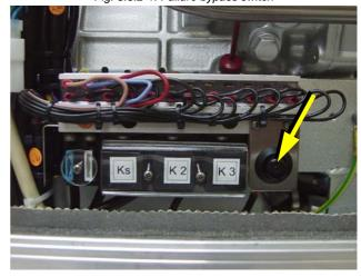
This period can be reduced by pushing the button on the front of the generator. The generator can be started by means of the remote control as long as the button is depressed. The switch/button bypasses any faults allowing the generator to run.
